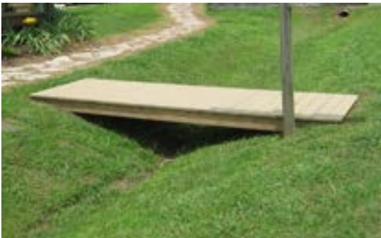
Bridge over swale.
