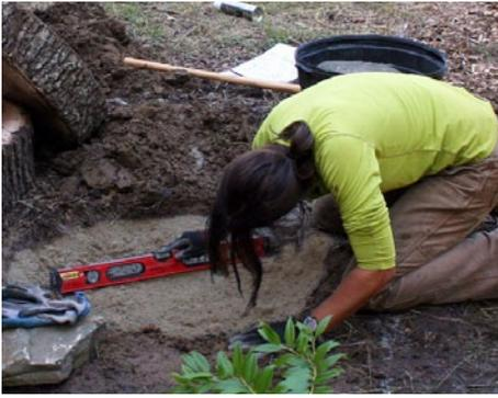
Figure 2 - Checking sand to make sure it is level.
