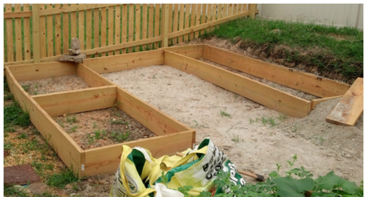
Building raised beds with 1" x 6" boards
