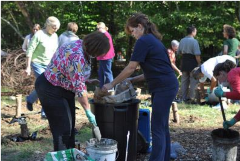
Mix concrete in buckets, and pour into prepared holes.
