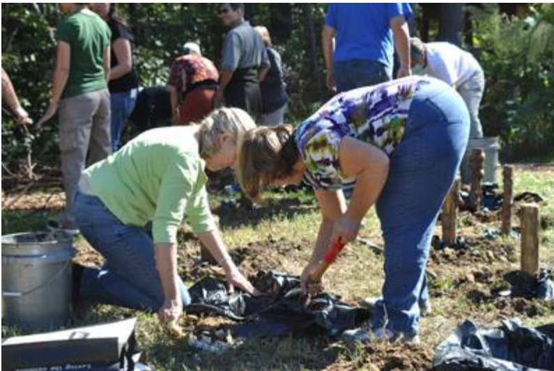
Pouring the concrete into the holes for the toadstool caps.
