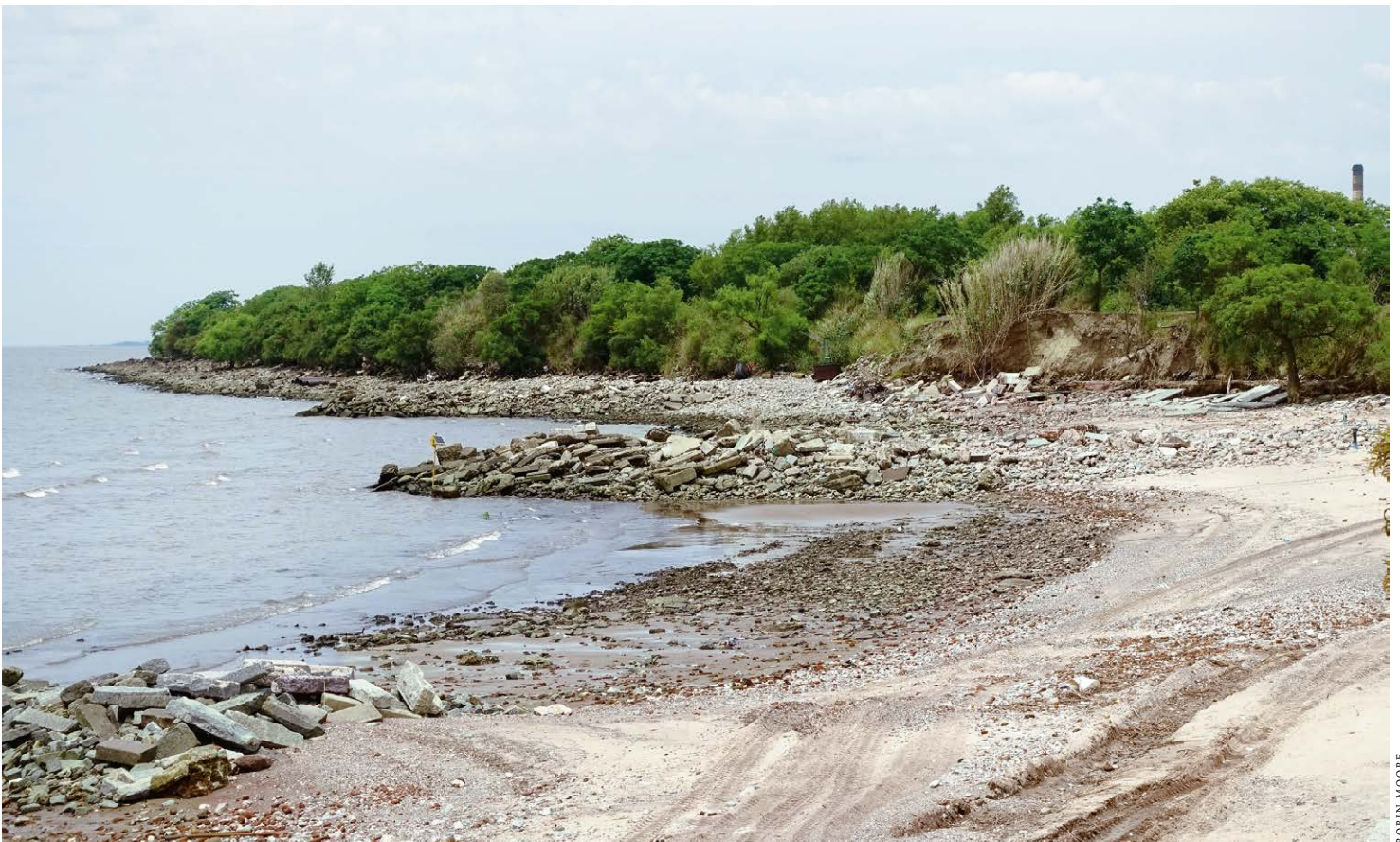
Figure 15 View looking south. The edge of the Reserva is armoured by the old demolition material. The concrete resists the wave action more effectively than the terracotta brick, which is decomposing more rapidly and changing the colour and chemical composition of the soil. The trees of the drier dike areas can be seen just upland, with an eroded bluff to the right.
