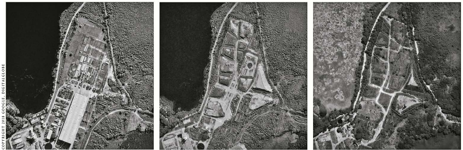
Figure 13 Earthworks on the brownfield. These time-lapse studies show the transformation of the Covimet factory brownfield site using 350,000 m 3 of excavated material. The slow forestation of the site can be seen from left (2004), to centre (2007), to right (2018). These processes of aggregation at industrial and ecological scales are characteristic of those that hatched the Reserva.
