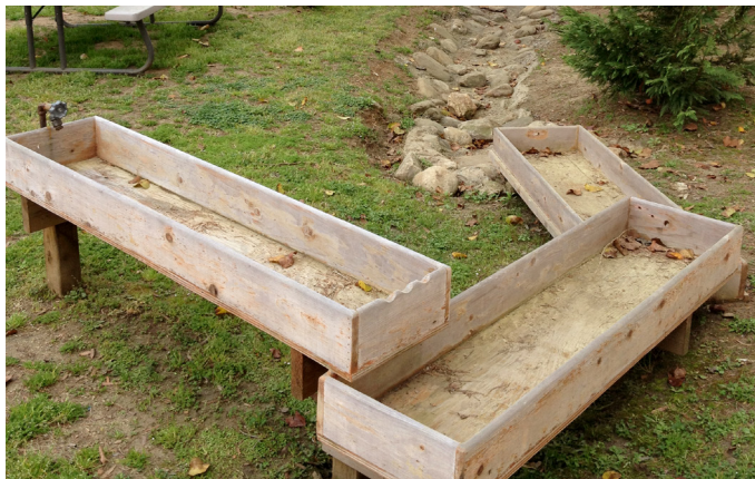
Raised, multi-level, interconnected water table. Water is supplied by an adjustable valve and exits into a dry stream bed converted from an eroding ditch.
