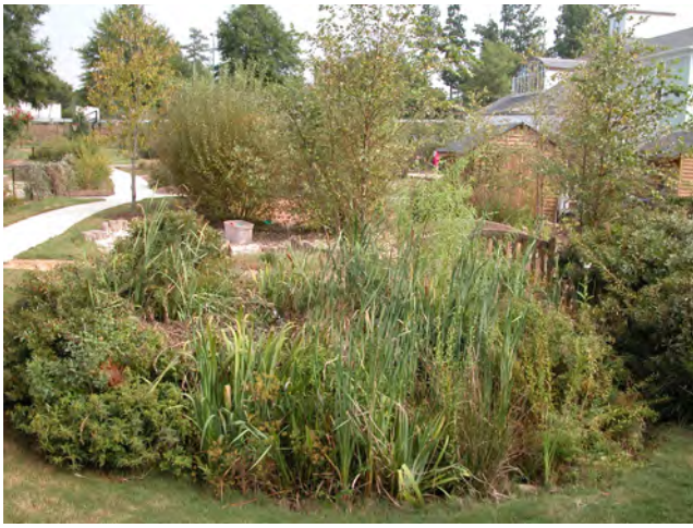
Figure 5. Vegetated swale ensures precipitation stays on site to recharge ground water to help sustain the local ecosystem. Courtesy of Robin Moore and Nilda Cosco
