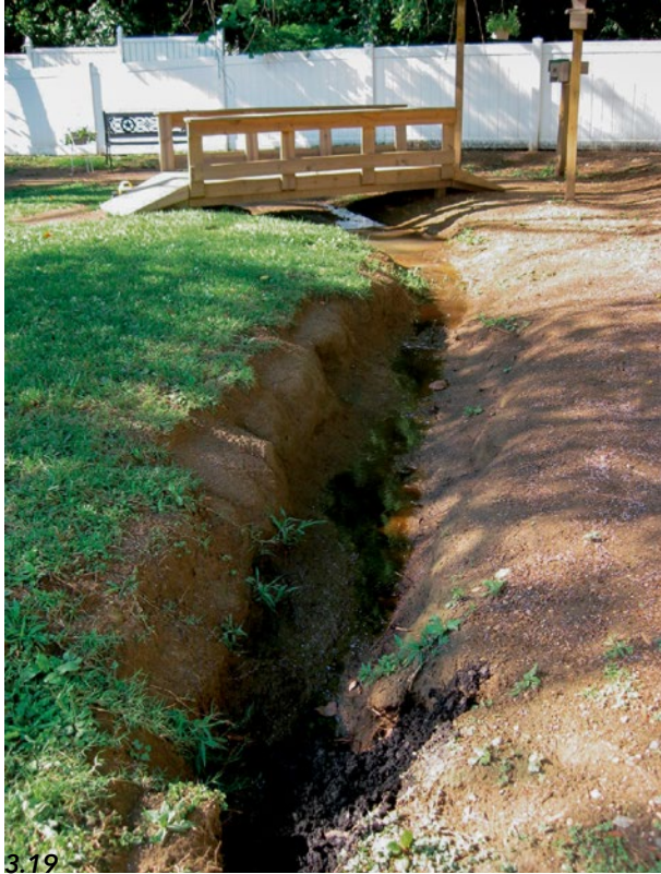
3.19 Gully erosion was a serious problem at this center before OLE renovation.
