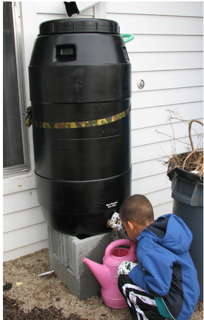
3. Barrel is secured by strap tied to wall.
