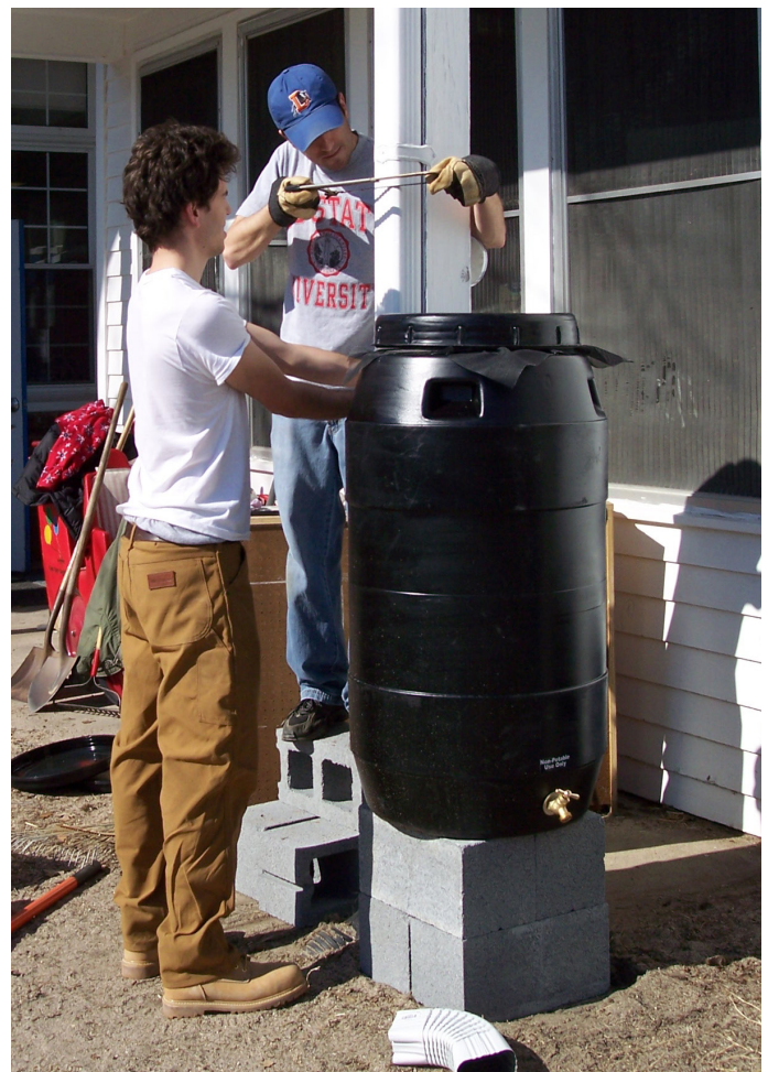
2. Installing a rain barrel on two layers of cinder blocks.
