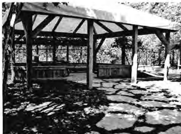
Figure 10-16: A naturalized outdoor classroom can immerse children’s learning processes in nature as well as reduce demands on interior, air-conditioned space. Roof covering is a translucent, waterproof, ultraviolet-light-resistant fabric. As they work, children can enjoy the experience of rain pouring down around them or the play of sunlight and shadow of foliage vibrating in the wind over their heads.
