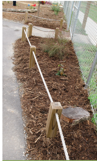
Barrier made from wooden posts and rope.
