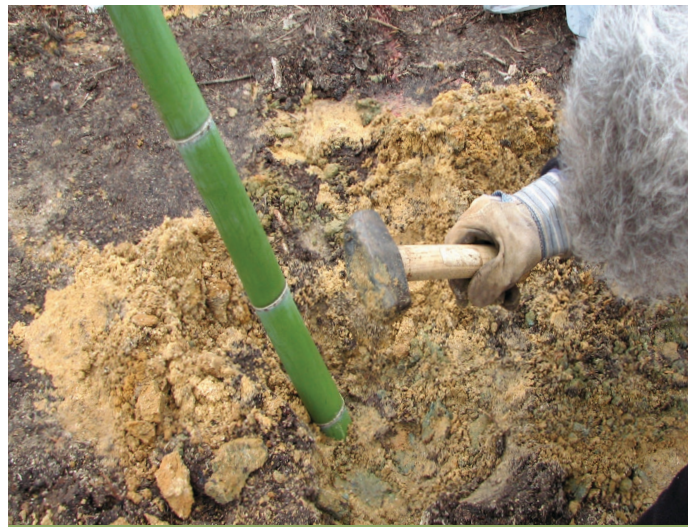
I. Fill holes and compact soil.
