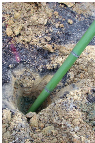
G. Place pole ends in holes
