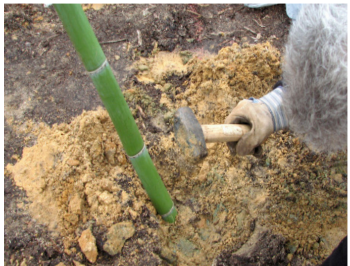
I. Fill holes and compact soil.
