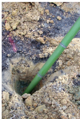
G. Place pole ends in holes
