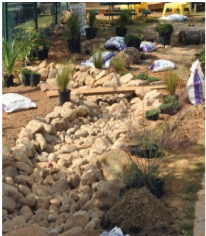
Installation of a dry creek bed prior to plant installation
