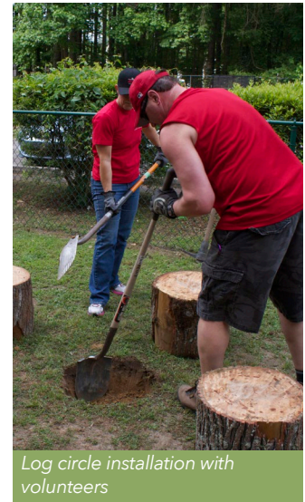
Hole depth should be approx. 1/3 log height plus 2" deep. Hole width should be log diameter plus 4"
